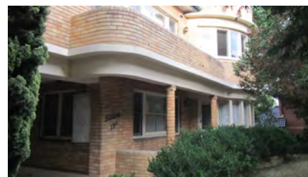
Photograph 14. Item I192 at 18A Cooper Street
