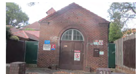
Photograph 15. State listed Electrical Substation
