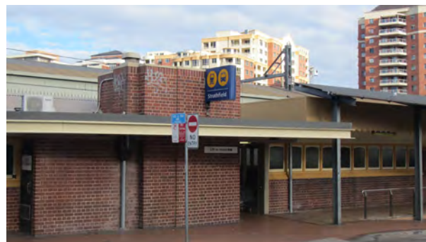
Photograph 10. Proximity to the Strathfield Train Station provides excellent opportunity for transit oriented development.
