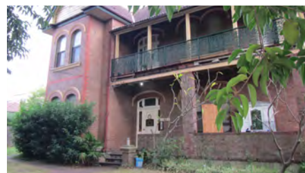
Photograph 13. Item I207 at 45 Wentworth Road
